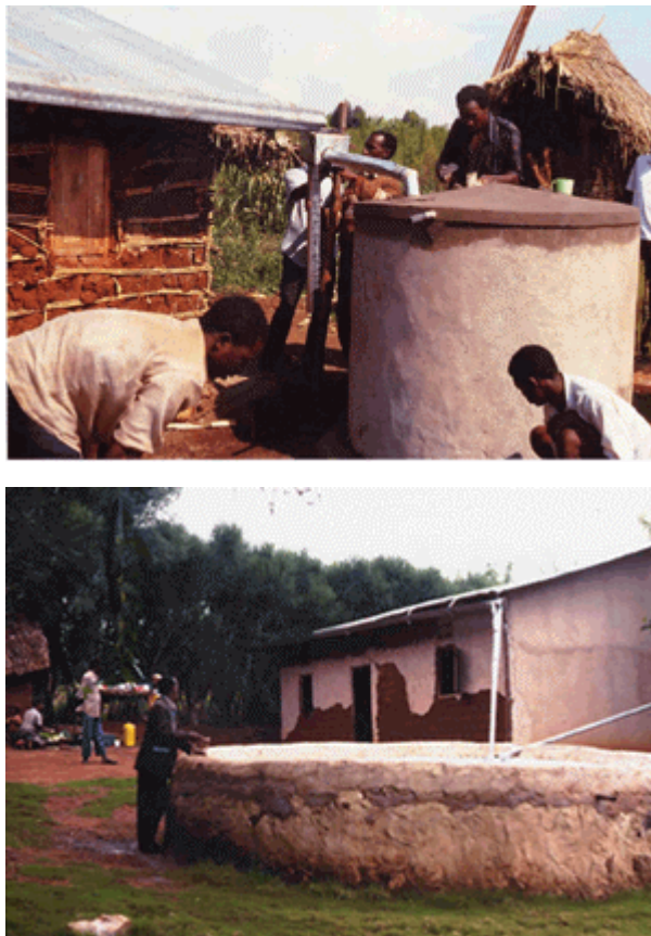
Rainwater tanks constructed by local builders called “fundis” in Kenya.
